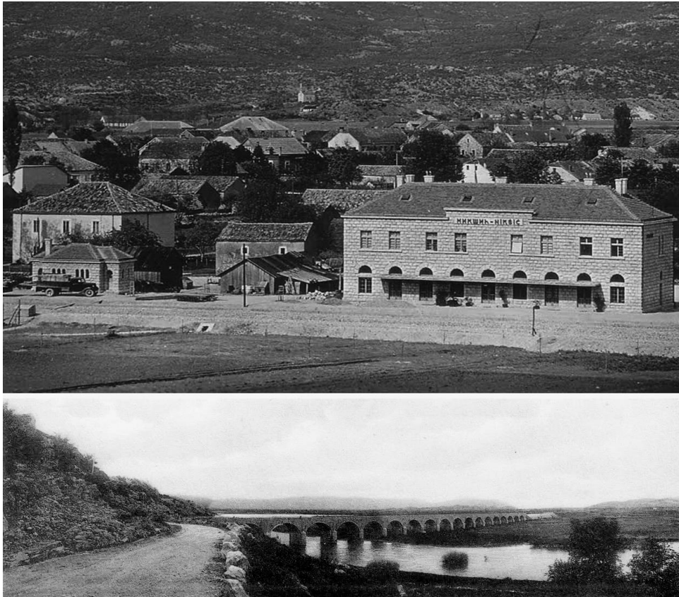
Figure 1. Panoramic view on Nikšić and the bridge (Carev most), year: 1955 (Source: State Archives of Montenegro)
